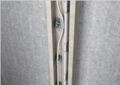
Vertical cable routing using cable brackets
